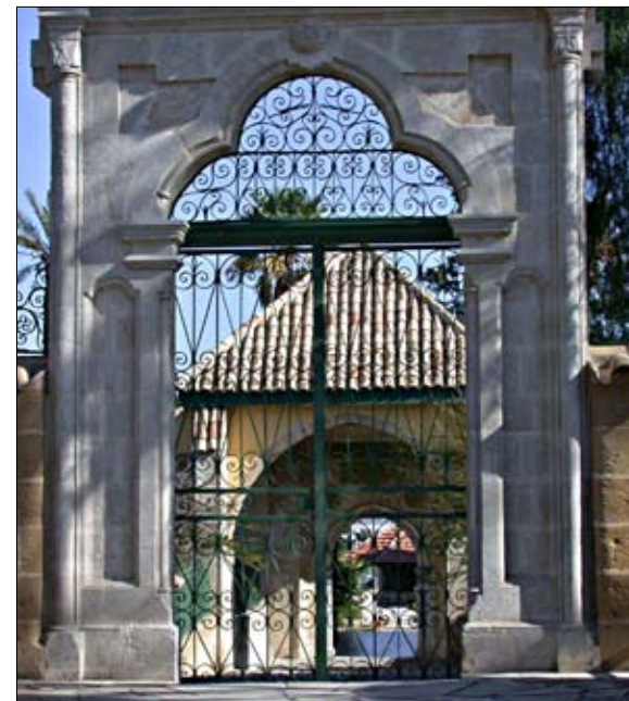
Outside door Hala Sultan Tekke, Larnaca. Photo H. Spohr
